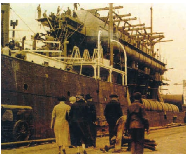
Claude’s final experiment with ocean thermal energy focused on retrofitting the Tunisie , above, into an ocean thermal ice factory with vacuum chambers and condensers. Off the coast of Rio de Janeiro, the Tunisie ran into problems with its long intake tube, a failure that finally bankrupted Claude.
