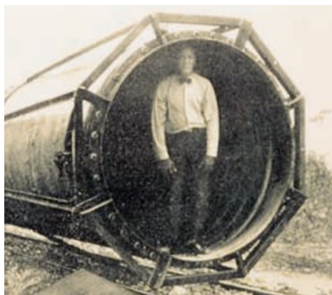
Deploying the 2,200-yard, cold water intake tube in Cuba, far left, proved the undoing of Claude, standing, left, inside the pipe. Storms, waves, and logistical problems encountered while laying the unwieldy and vulnerable pipe, above, sank Claude’s dream to harvest energy from the ocean.
