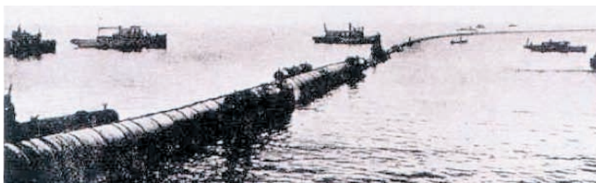
Deploying the 2,200-yard, cold water intake tube in Cuba, far left, proved the undoing of Claude, standing, left, inside the pipe. Storms, waves, and logistical problems encountered while laying the unwieldy and vulnerable pipe, above, sank Claude’s dream to harvest energy from the ocean.
